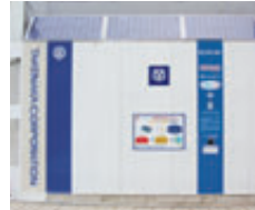
Solar panels, LED light guide panels, and environmental bulletin board on the temporary fence
