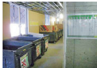
Locating multiple separation yards when and where appropriate depending on the progress of the construction work
