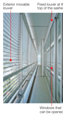
Figure 1. Exterior appearance adapting to the environment
