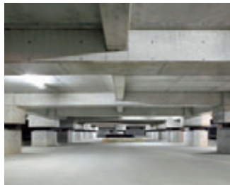
Quake-absorbing system under the stereobate
