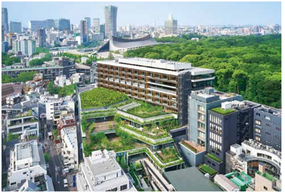
Cool prevailing winds from the Meiji Shrine blow through the Passage and greenery of the outdoor terrace, which has a temperature-lowering effect on the surrounding blocks.
