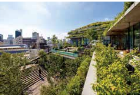
By providing a verdant stepped terrace that recreates the Genjiyama Hill of the Edo period, a flourishing environment overlooking the cityscape opens toward the city.
