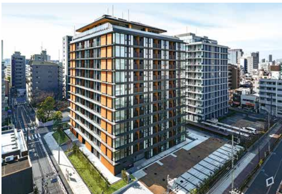
A 12-story wooden building was realized by developing many next-generation wooden construction technologies that enable wooden buildings in urban areas.
