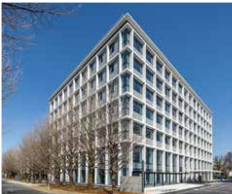
The exterior was designed with grid fins symbolizing "logic" and "harmony" to optimize the lighting environment and reduce the solar radiation load.
