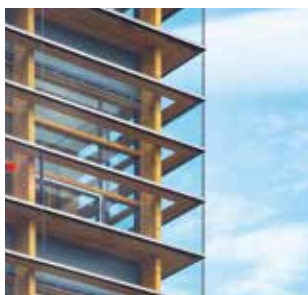
A double skin facade supported by laminated wood reduces the environmental load, and the quality of the wood can also be felt from the outside.
