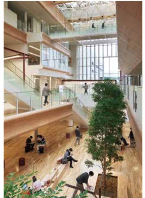
Wood harvested by students was used for reinforcing top lights and for furniture.
