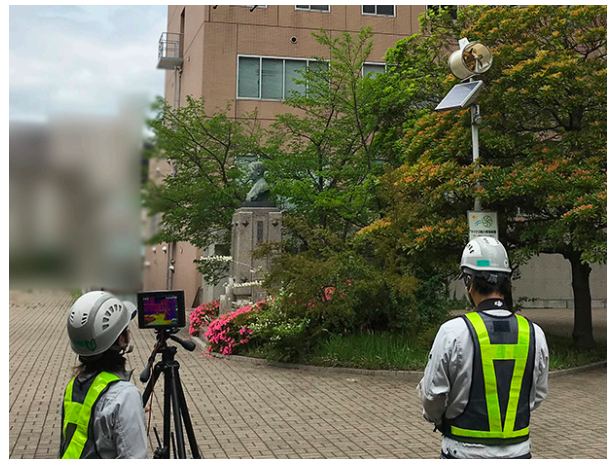
Using a drone to inspect exterior wall tiles (with infrared cameras)
