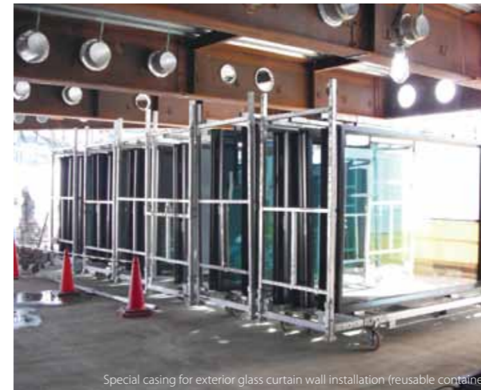
Special casing for exterior glass curtain wall installation (reusable container)
