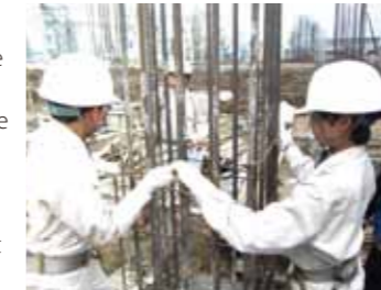
Experience in tying reinforcement rods
