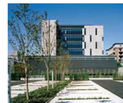
Takenako Corporation Tokyo Main Office The new main office pursues self reliance as a zero energy building through such means as capturing natural light, harnessing wind for use in air conditioning and solar power generation.
