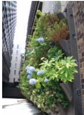
Wall greening of the Mido Building
