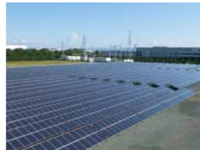
Mega solar power plant construction
