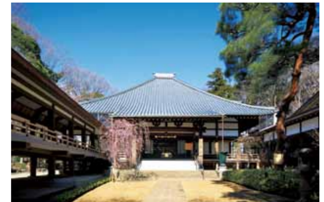
Horinouchi Myohoji Temple Hondo (Main Hall) The Main Hall of Myohoji Temple at Horinouchi, constructed in 1819, was restored to extend its service for many more years. Aseismic reinforcement was installed using a "zinc aluminum damper" with superplastic capacity. The restoration, including interior and exterior renovation, landscaping design, roof retiling, and air-conditioning and lighting system installation, was conducted while maintaining the hall's character to the greatest extent possible, thus recapturing the charm of this ancient temple. Renovation design and construction: Takenaka Corporation
