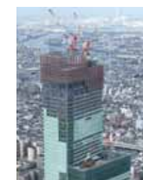
Slide cover construction
