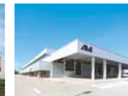
Aisin AI (Thailand) No. 3 Factory 2 (Thailand, 2013)
