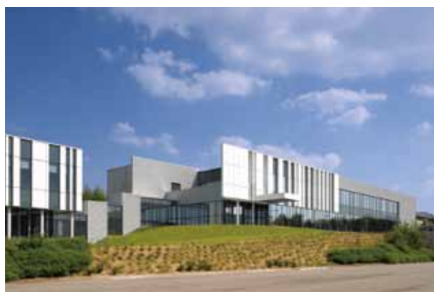
GC Europe Head Office Building (Belgium, 2013)
