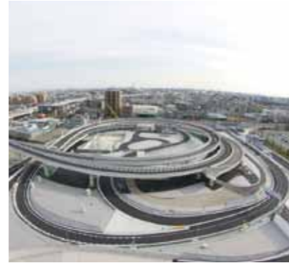
Daishi Junction on the Kawasaki section of the Tokyo Metropolitan Expressway
