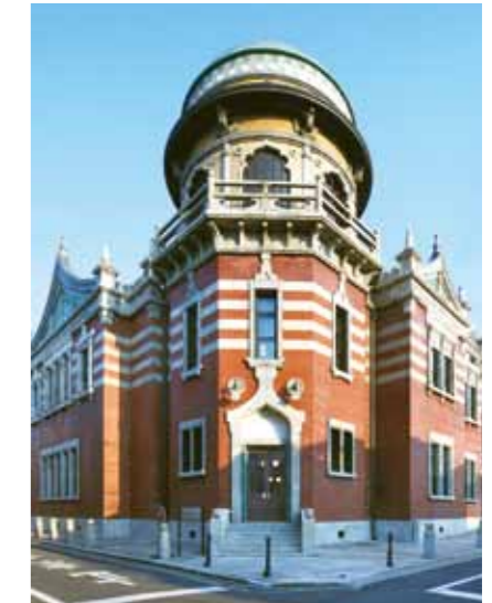
Restoration of Dendo-in of Nishi Hongwanji Temple Constructed by Takenaka in 1912, Dendo-in Nishi Hongwanji Temple's was restored for the 750th Great Annual Memorial Service for the Buddhist monk Shinran. Its seismic performance was enhanced without damaging the external walls, and its character of a century ago was resurrected. Recipient: 22nd BELCA Award. Restoration design and construction: Takenaka Corporation
