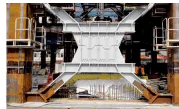
New steel alloy system swinging damper
