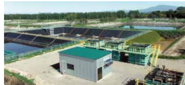
Odor-reduction measures implemented at a starch plant
