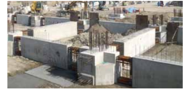
PC foundation construction
