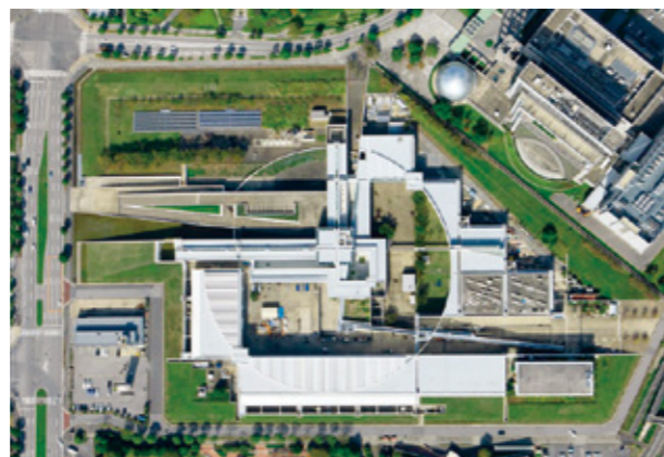
Exterior view of the Takenaka Research and Development Institute
