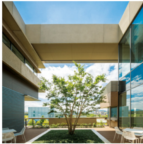
This west-facing terrace is located on the third floor. From it you can see the National Diet Library's Kansai-kan in the front.
