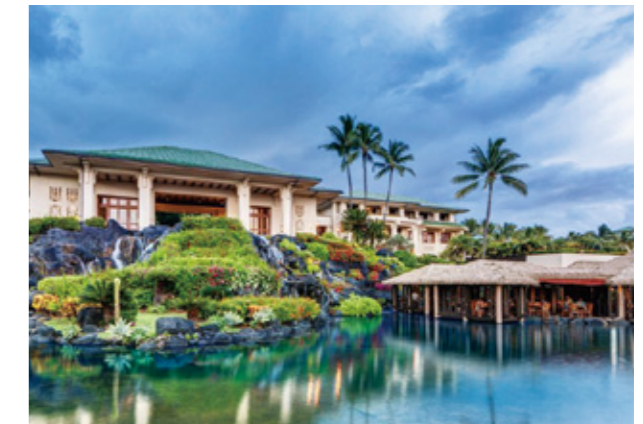
Design: Wimberly Allison Tong and Goo Construction: Takenaka Corporation (U.S.A.)
