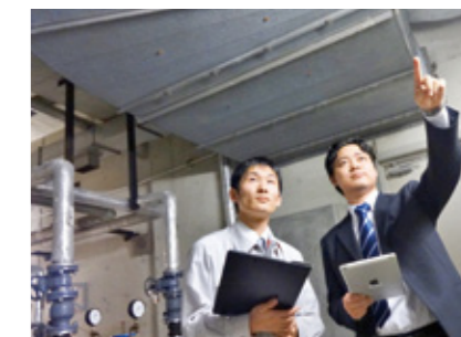
Facilities check using mobile terminals
