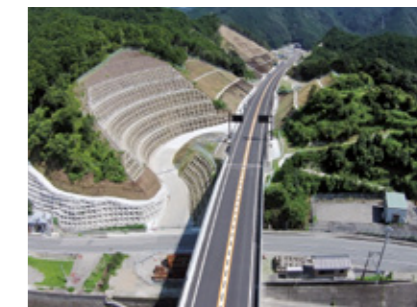
Kinki Expressway Kise Line Tachino zone improvement work
