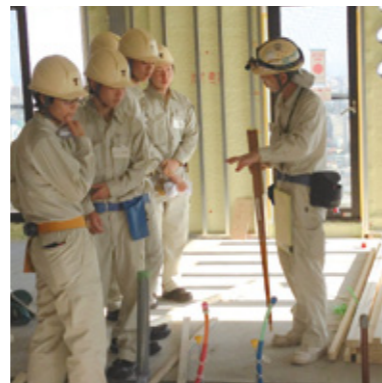
Training at a construction site
