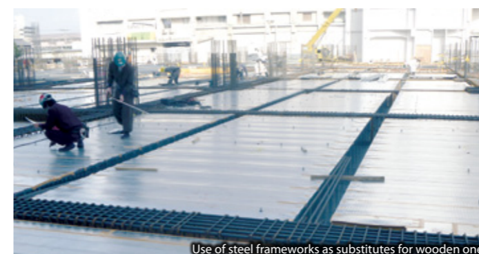
Use of steel frameworks as substitutes for wooden ones
