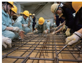
Students practicing ferro-concrete reinforcement
