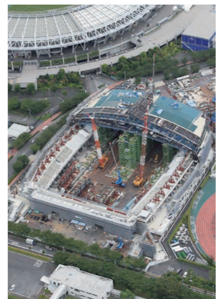
Roof of the arena under construction
