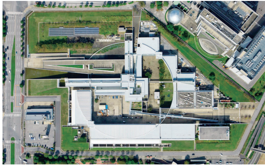
Exterior view of the Takenaka Research and Development Institute
