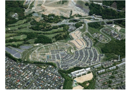
Land formation work of the Aigawa land readjustment project
