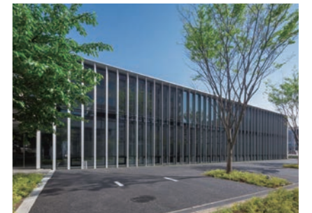
Renovation work into a ZEB for Takenaka's Higashi Kanto Branch
