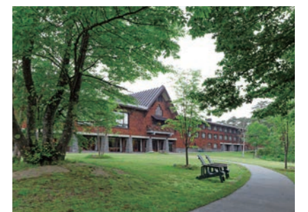
Hotel seen from the courtyard
