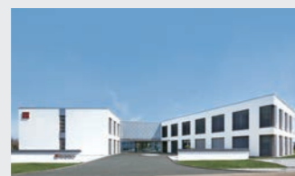
Takasago Europe New Office & Conference Building (Germany, 2015)
