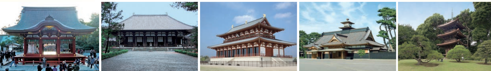
Tsurugaoka-hachimangu Maiden (Seismic reinforcement in 2006)
