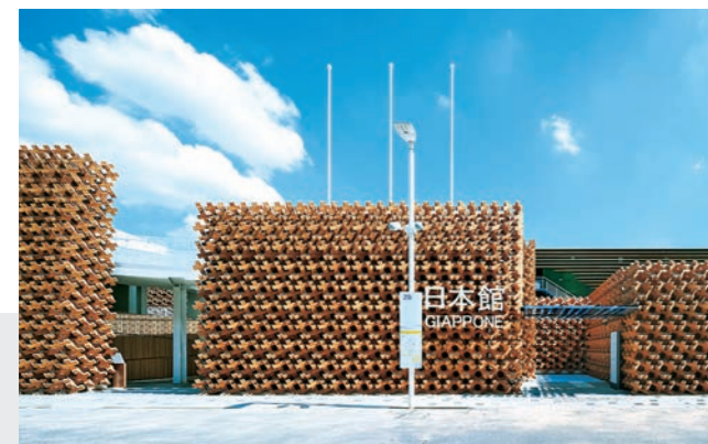
Expo 2015 Milano Japan Pavilion (Italy, 2015)
