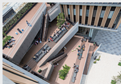
The "step terraces" guide student movements and offer a resting area with views of surrounding greenery and Mount Fuji. They also function to bring outside air into the buildings.
