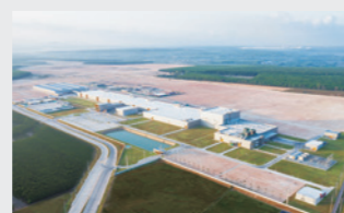
Continental Tyre Thailand New Plant (Thailand, 2018)
