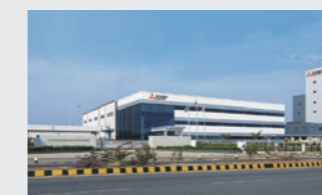
Mitsubishi Elevator India New Factory (India, 2016)
