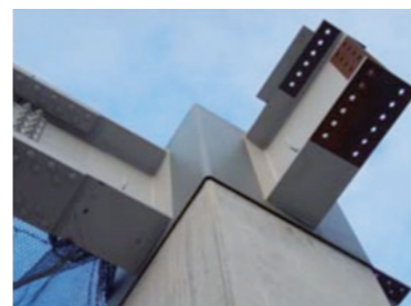
Beam-column connection in the T-ReCS Method
