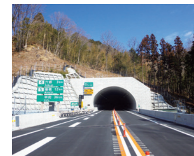
Chubu Odan Expressway Shiroyama Tunnel Project
