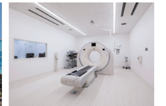
CT simulation room installed with RadBoard-X
