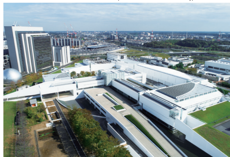
Aerial view of the Takenaka Research and Development Institute
