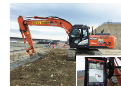
Machine guidance backhoe
