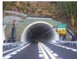
East Neguma Tunnel, Chubu-Odan Expressway
