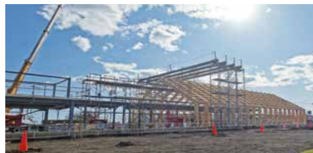
Building structural frame made of larch from Hokkaido
