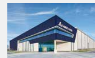
Sanko Gosei Gujarat New Factory (India, 2018)
