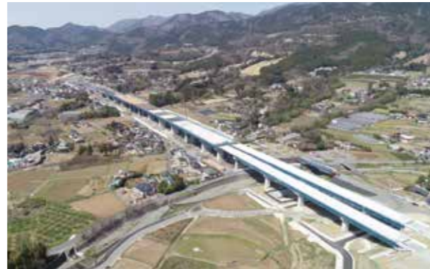
Kuzuha River Bridge, Shin-Tomei Expressway
