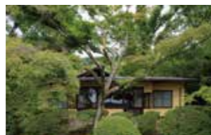
Exterior of the main building after completion of restoration work
