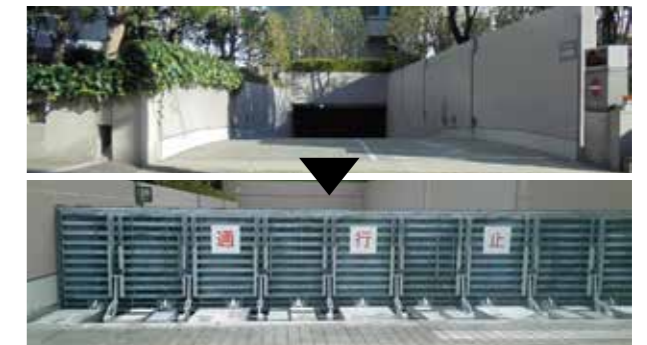
Flood shutter installation
