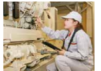
Power generator inspection
