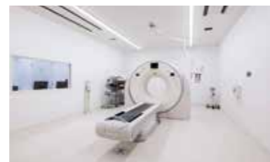
CT simulation room installed with RadBoard-X
