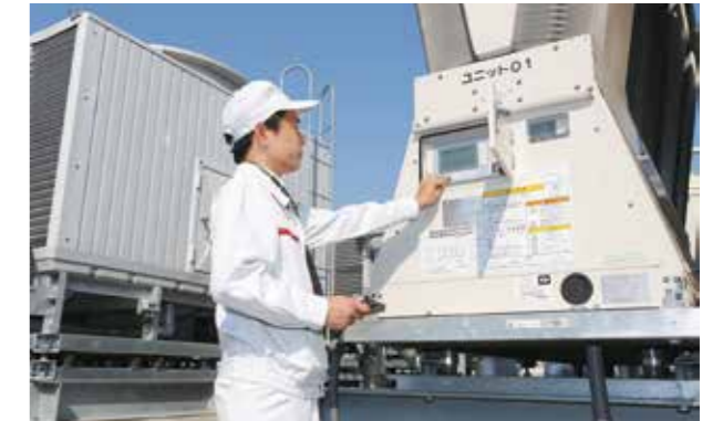
Rooftop facility inspection
