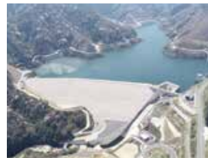
Oitagawa Dam construction
