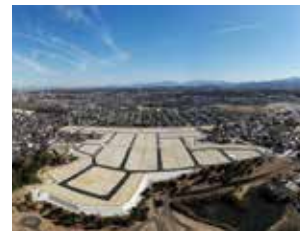
Construction in 3-chome Hatsugano, Izumi city, Osaka
