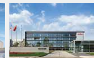
Wuxi Murata Electronics Second Factory (China, 2020)
