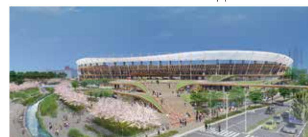
Paloma Mizuho Stadium, integrated with the adjacent park
