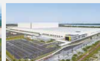
IKEA Distribution Centre Port Klang (Malaysia, 2020)
