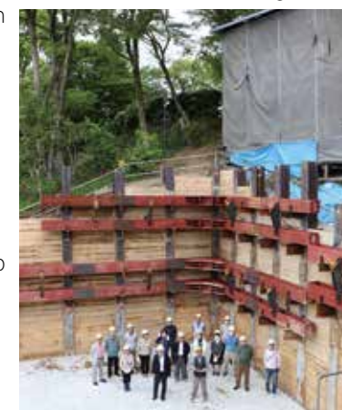
Underground water storage tank, pump room and earth retaining work
