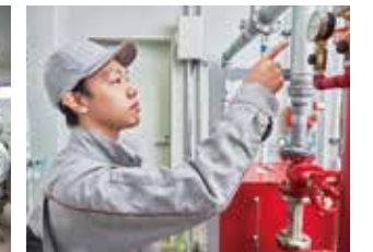
Inspecting fire extinguishing equipment
