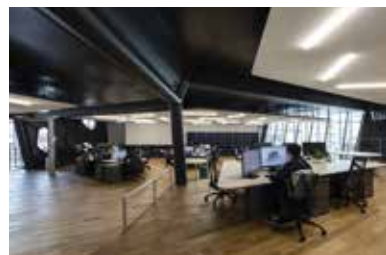
The workspace interior is expressed with steel used not only for beams and columns but also for the slab (floor).
