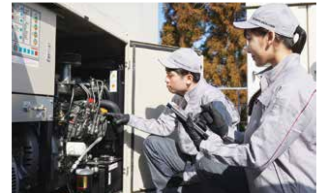
Inspecting an emergency power generator
