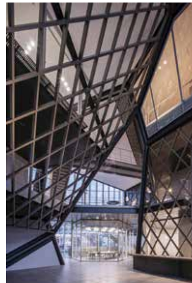
The employee entrance to the complex steel frame structure is also a space for interaction among coworkers entering the factory.
