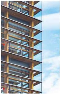
The double skin facade supported with laminated wood has a low environmental impact and gives the impression of wood from the outside.
