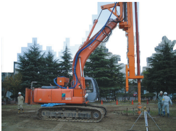
Photo 1 DCM-e工法での施工機械 Mixing machine for DCM-e method
