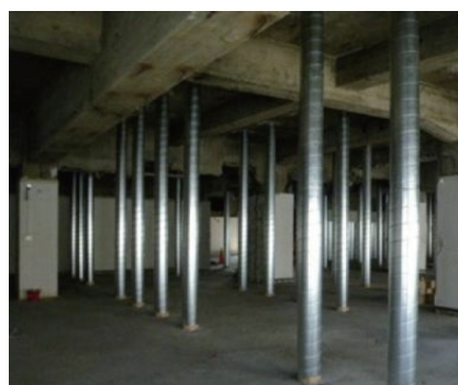
Photo 2 補強サポート設置状況 Situation of reinforcement support
