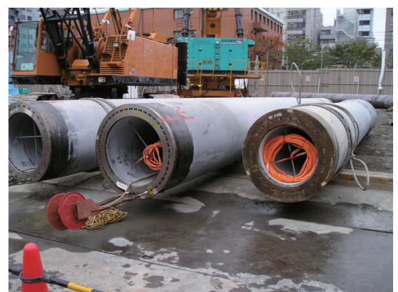
Photo 4 Instrumented PHC piles
