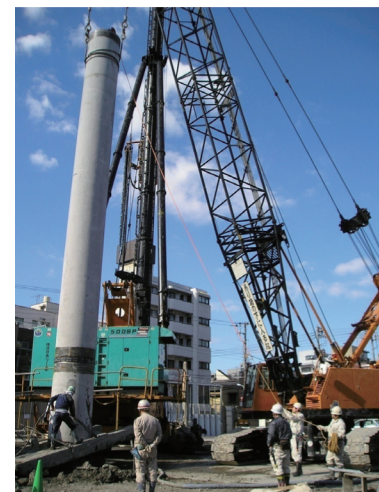
Photo 3 Construction of PHC piles (1.2 m in diameter)
