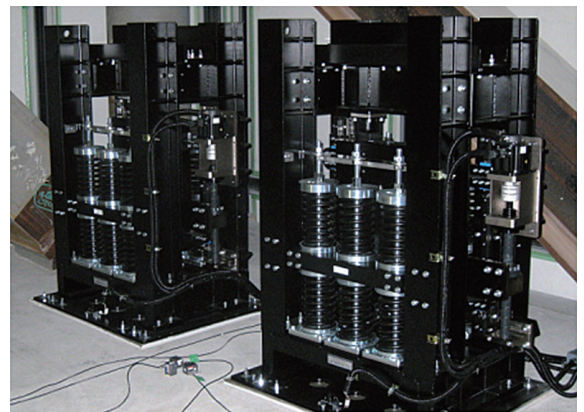
Photo 4 受振側の建物内にHMDを設置した例 Example of HMD installed in the building on the receiving side
