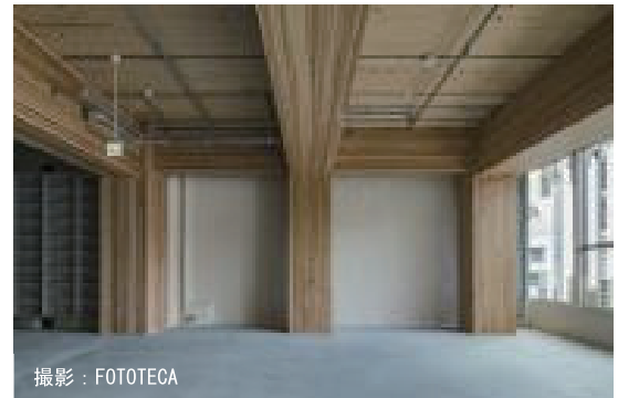
Photo 2.3 HULIC & New GINZA 8 (左: 外観 右: CLT合成床) (Exterior and CLT composite slab)
