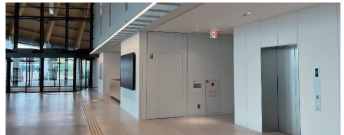
Photo 4 出火場所に応じて進入禁止を表示する誘導灯の設置状況 Installation status of emergency exit sign displaying entry prohibition according to fire location
