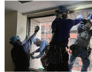
Removing glass panels from a demolition site.
