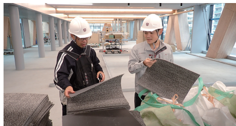
Reusing tile carpets originally destined for disposal in a new construction project
