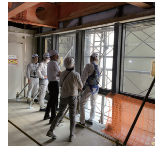
Examining the dismantling procedure of aluminum sashes in an existing building.
