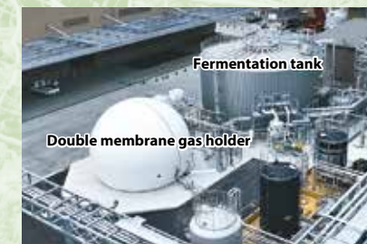
Raw material input capacity (design): 50t/day Production wastewater inflow capacity (design): 750m 3 /day
