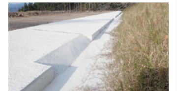
Waterway with slopes to protect small creatures
