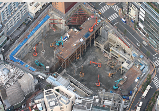
Birds-eye-view of the underground work utilizing an existing building frame
