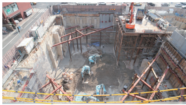
Underground work utilizing an existing solid structure
