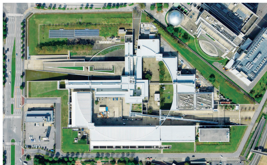
Aerial view of the Takenaka Research and Development Institute
