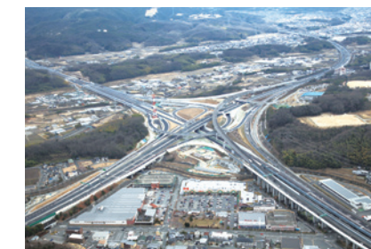
SHIN-MEISHIN EXPRESSWAY (courtesy of West Nippon Expressway Co., Ltd.)
