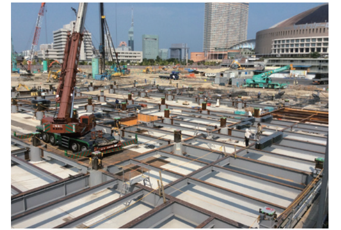
Usage of steel foundation and steel footings, and flattened work floor
