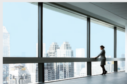
The large unit curtain wall with its outstanding environmental performance has created a workspace with a sense of openness and an outstanding view.
