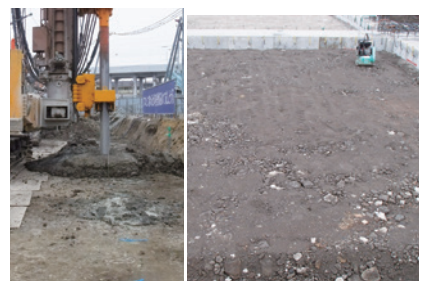
Recycling construction sludge mixed into foundation soil
