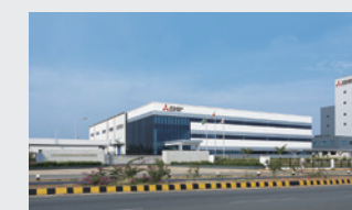
Mitsubishi Elevator India New Factory (India, 2016)
