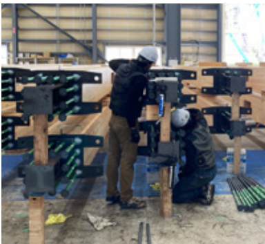
Preassembly at off-site logistics center for EXPO 2025 construction in Osaka, Kansai
