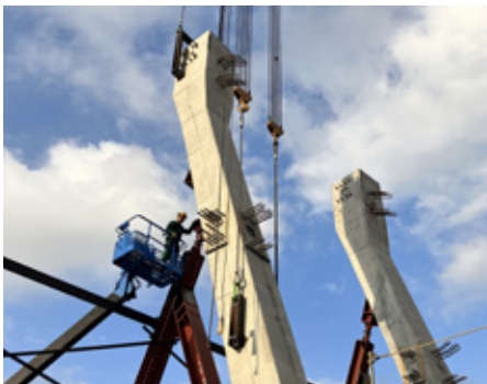
Using precast concrete for the slanted columns considerably reduces the amount of on-site work.
