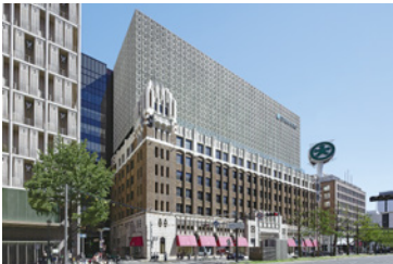
Main Building of Daimaru Shinsaibashi Store Completed: Phase I in 1922 to Phase VI in 1933 / Renovated: 2019 We restored and preserved the original symbolic exterior wall, and reused interior parts to restore the store space.
