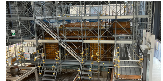
Reinforced concrete mock-up
