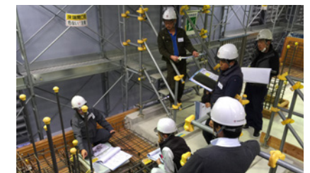
Reinforcement inspection training with a subcontractor
