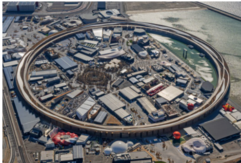
2025 Expo 2025 Osaka, Kansai, Japan's Grand Ring (West Construction Area)
