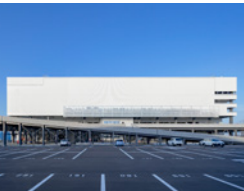
Logistics fund: logistics facility in Ogimachi, Sendai City
