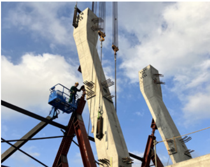
Use of precast concrete for slanted columns significantly reduced on-site work
