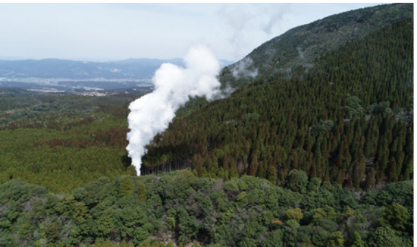
Geothermal power generation
