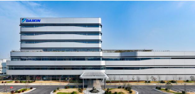
DAIKIN Suzhou R&D Center (China, 2025)
