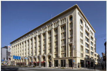
Takashimaya East Building Completed: 1940 / Renovated: 2019 We renovated the department store building, known as “the best in the Orient,” into a complex that includes a hotel and museum.
