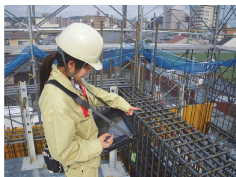
Photo 2 配筋検査状況 Field inspection of rebar by RCS
